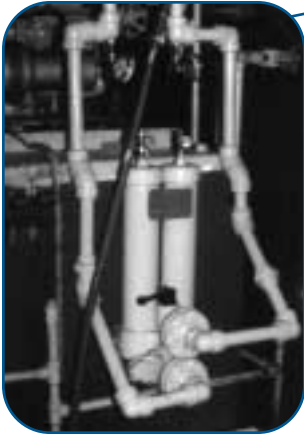
Pall 8950 duplex filter assembly in use on a seal oil system
